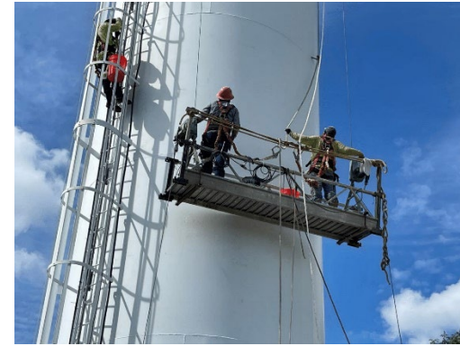
The Wheatley tank gets cleaned and painted, inside and out.
