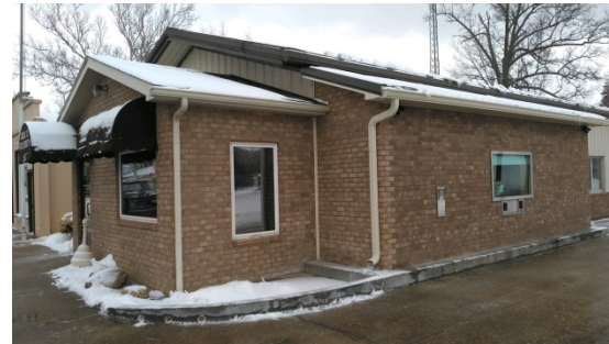
Carroll County Water turns a bad situation into something positive for our customers! We built a drive up pay/service window and a drive up overnight drop box.
