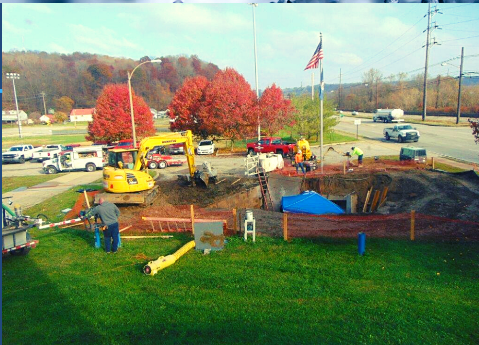
Above: The Water Treatment Plant receives an upgrade! This is a picture of contractors working to install the new finished water meter at the WTP. The new meter allows us to measure consumption more accurately yielding more efficient operation. This is part of the ongoing SCADA upgrade project at the WTP.
