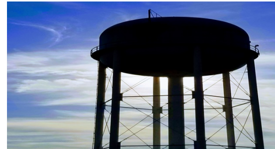
Most people don't realize this is one of your most important structures in your community.
