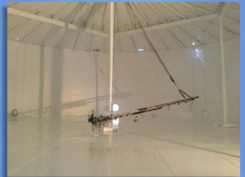
Figure 3: Tank Interior After
